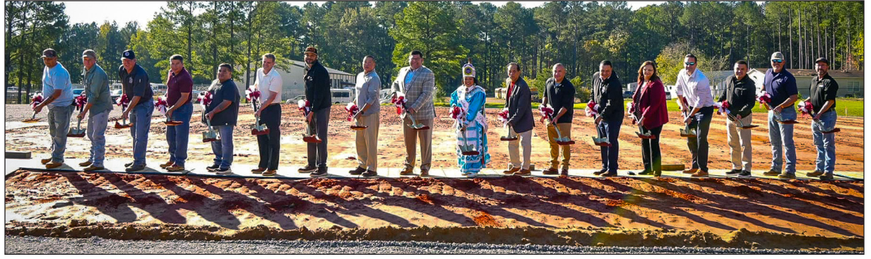
Ground was broken for a new Broadband Building to be constructed near the Office of Construction Management in the Pearl River community. The building is expected to be completed in Fall 2025.
