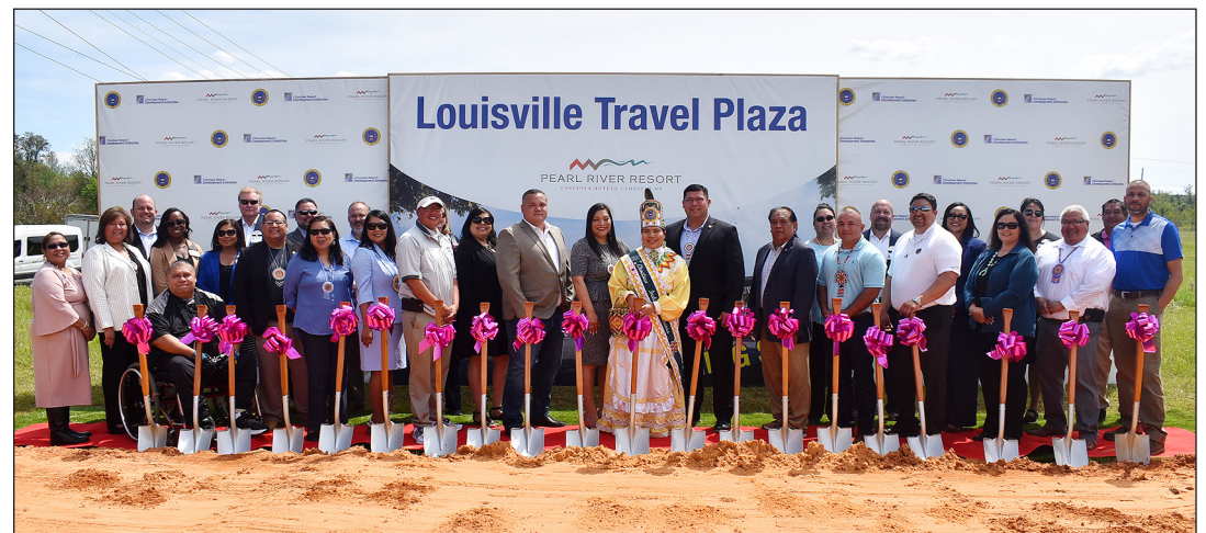
Officials with the Mississippi Band of Choctaw Indians and Pearl River Resort break ground for the Louisville Travel Plaza project on Wednesday, April 12. The target opening is slated for the Summer of 2024.
